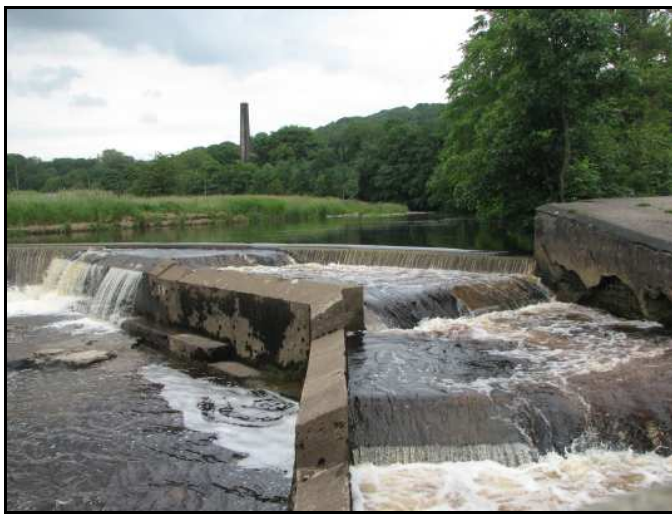
Figure 6. Pass at 1.78m 3 /s. (Q50)
