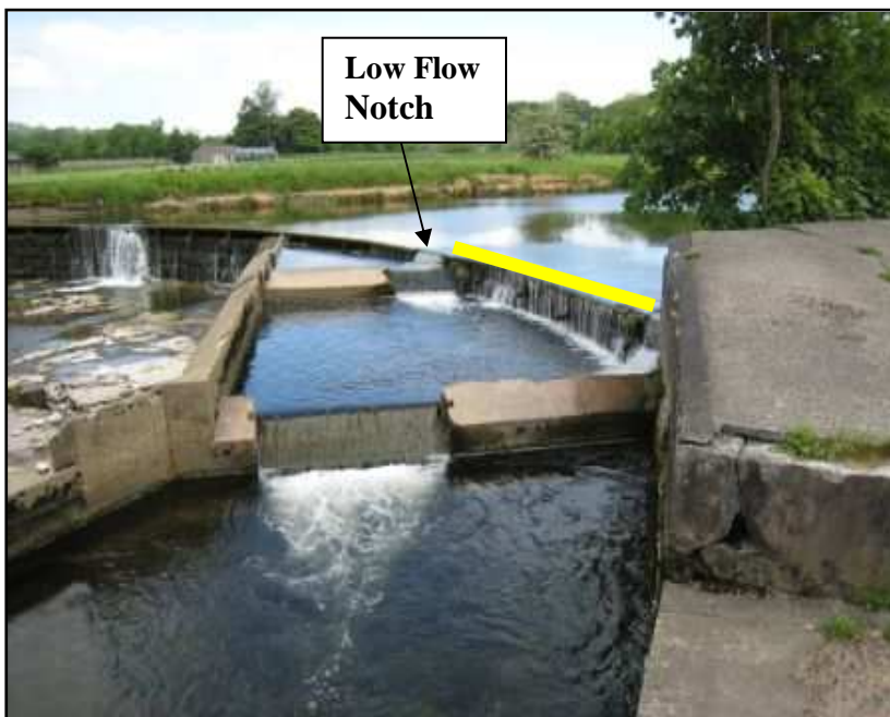
Figure10a. Modifications to reduce flow in pass and prevent fish being drawn into leat.
