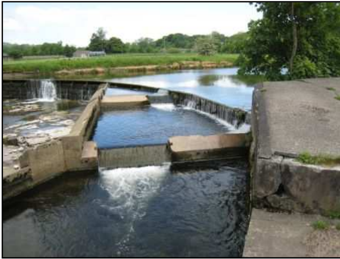
Figure 4. Pass at 0.336 m 3 /s, just below Q90
