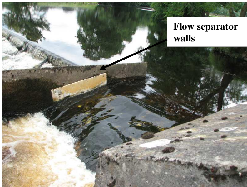
Figure 10. Fish pass at Locks weir
